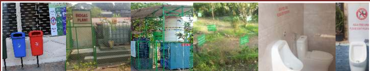
BIO-DIGESTER FOR WASTE MANAGEMENT, WATER MANAGEMENT WITH STP, WATERLESS URINALS & DRIP IRRIGATION
